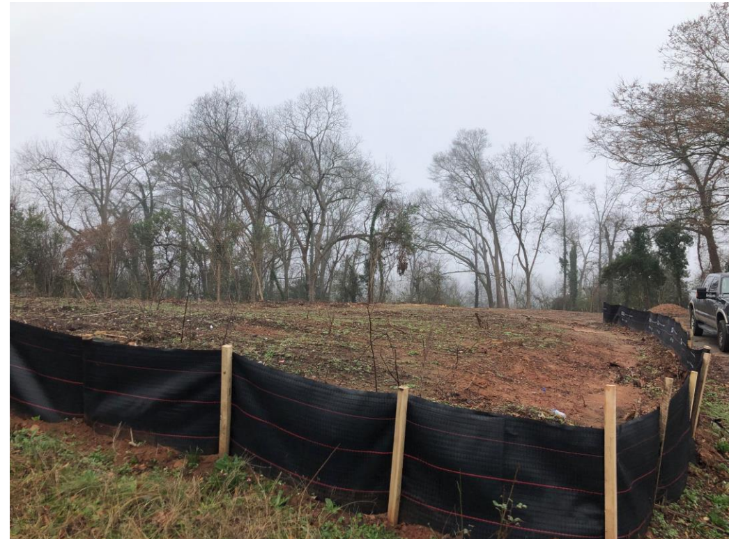
Subject properties with debris removed
