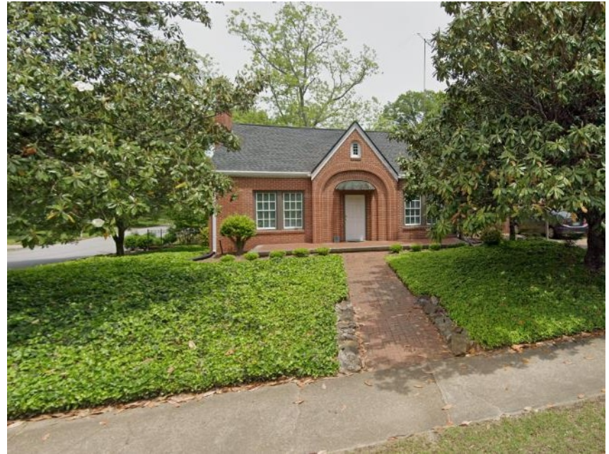
Adjacent neighbor to the south at 53 Clark Street
