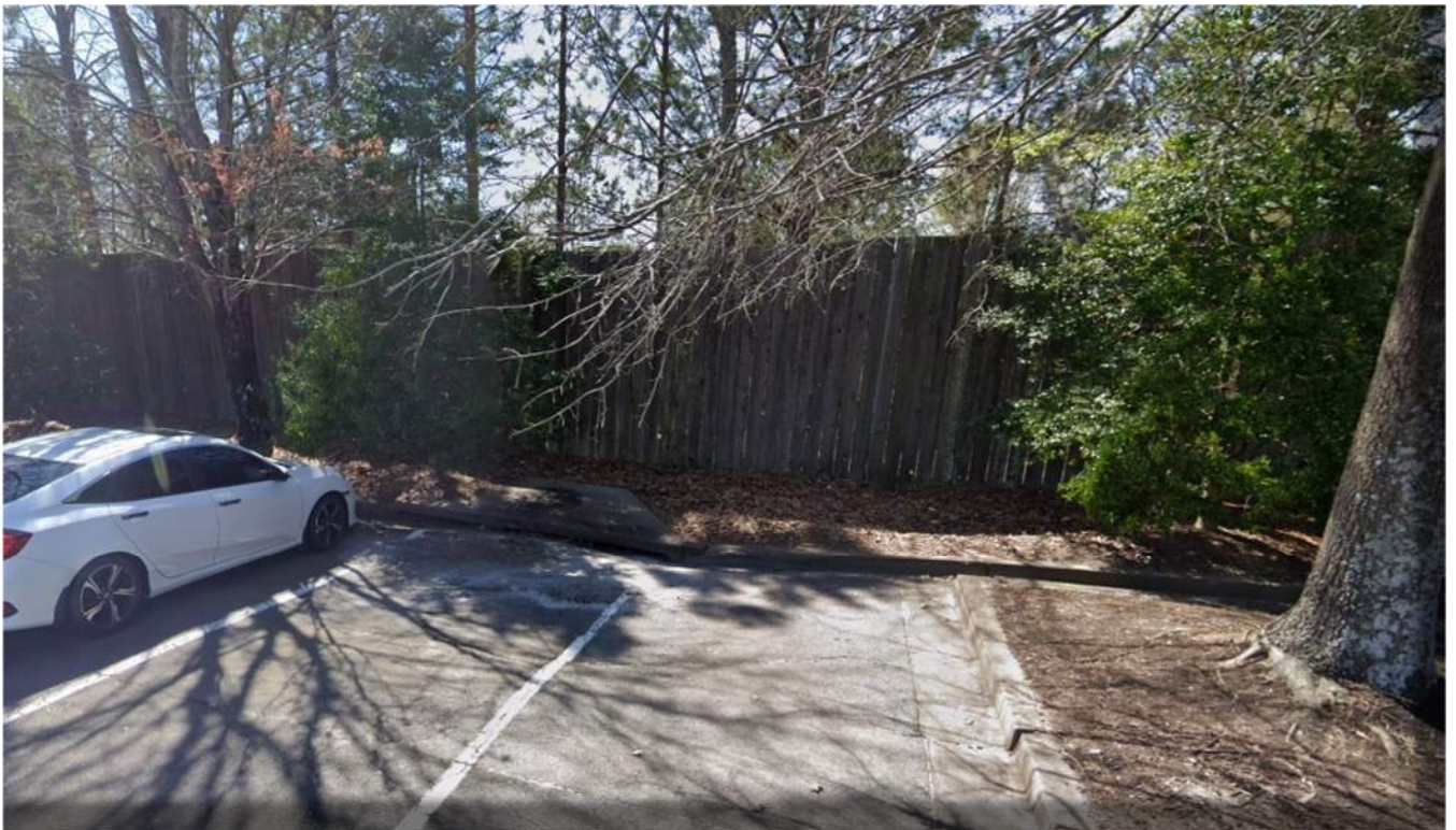
Figure 4: Detention Pond Fencing in shopping center
