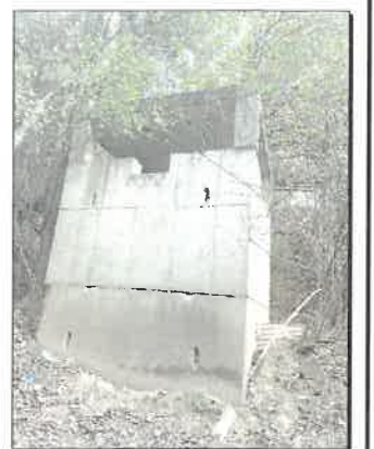
③ SIDE VIEW WESTERN OCS
