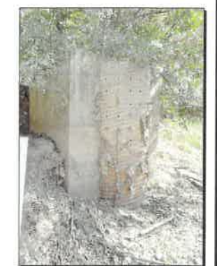
① FRONT VIEW NORTH WESTERN OCS
