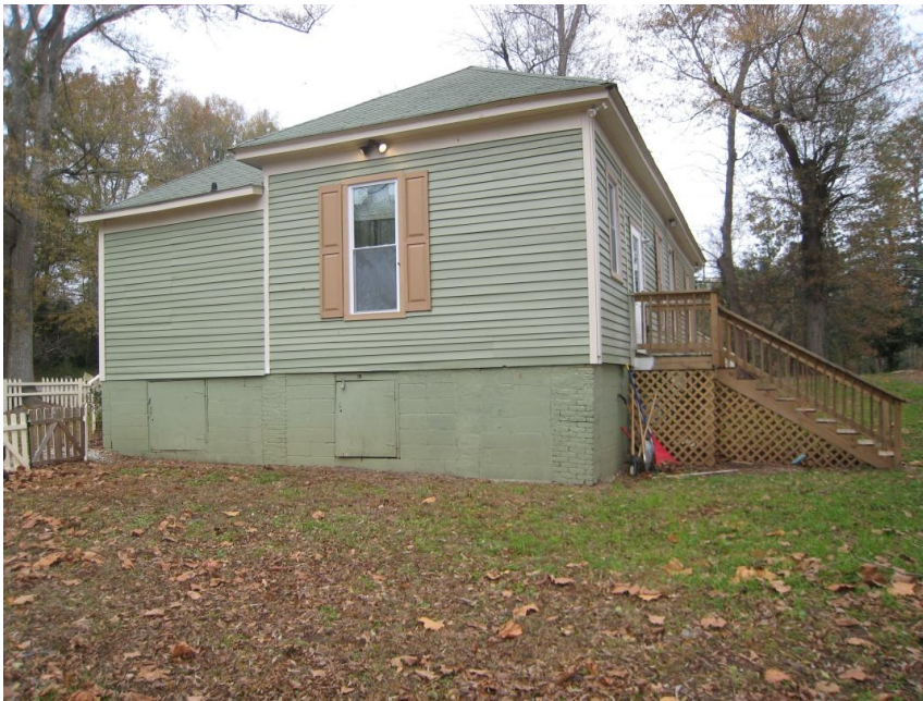
View of rear façade of existing home on subject property
