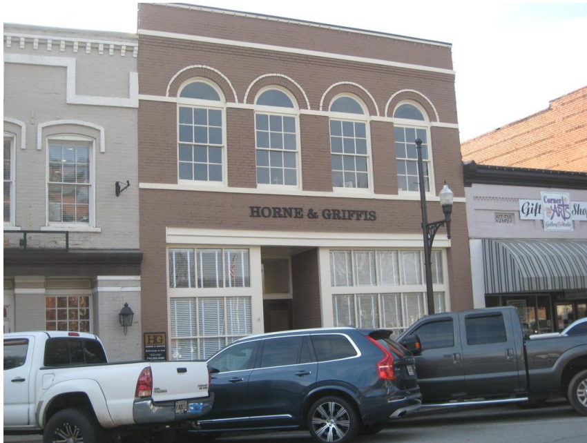
View of adjacent property to the west (32 South Court Square – Horne & Griffis building)
