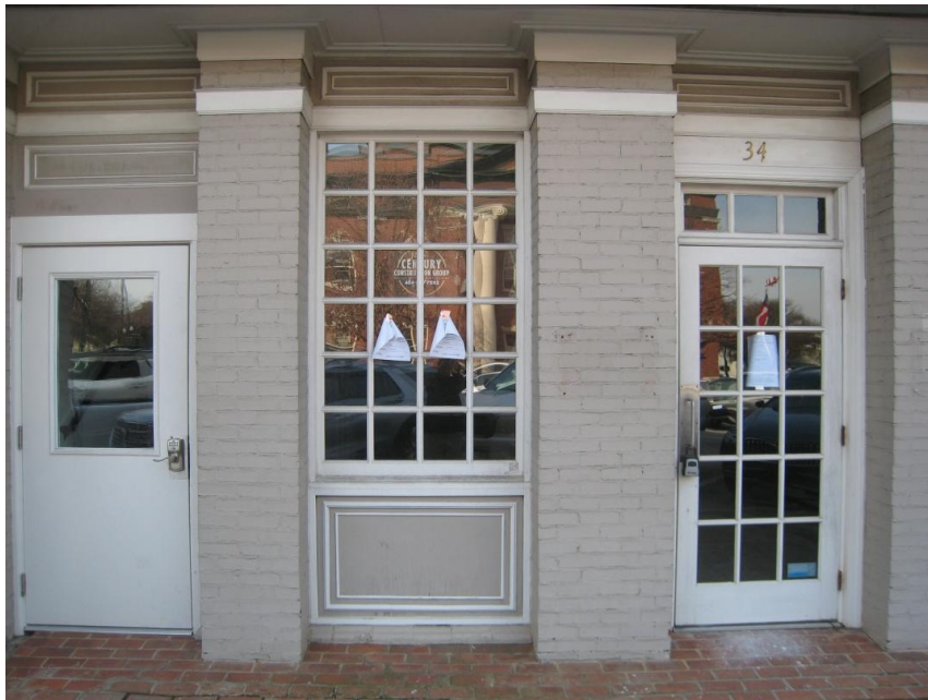
Current View of Subject Property's Ground Floor
