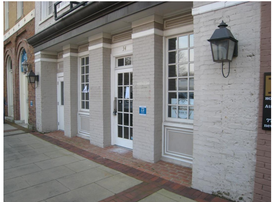
Current View of Subject Property's Ground Floor (with the lantern columns marking the edges)
