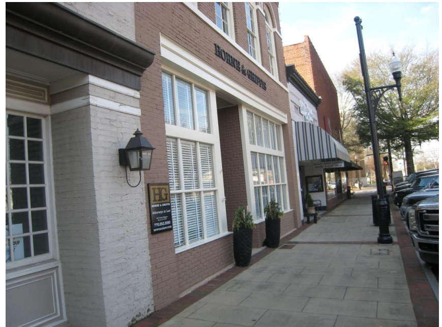
Ground-level view of building to the west (32 South Court Square – Horne & Griffis building)
