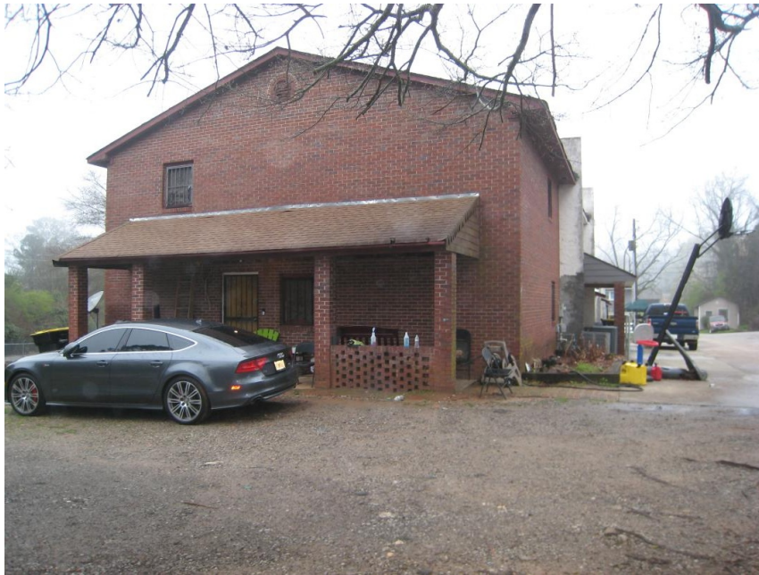
View of adjacent residential units at 34 Haynie Street (looking from the Subject Property)
