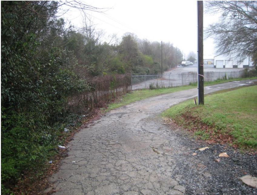
View of Haynie Street (with 226 Greenville Street in the background)
