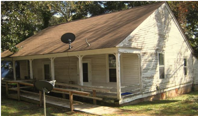
Before and After Pictures
