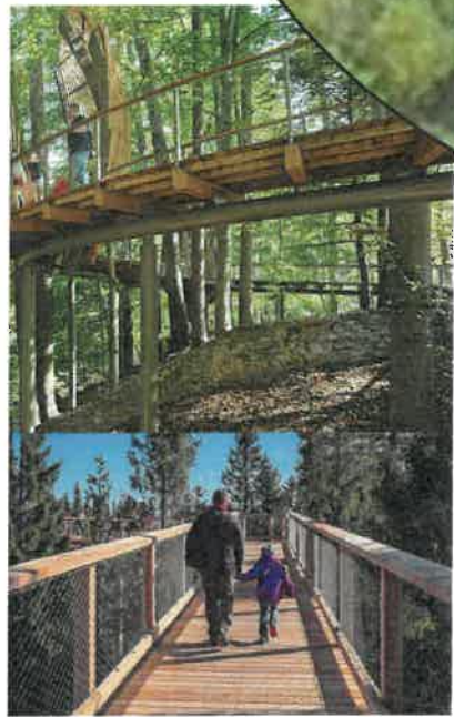
Accessible Elevated Boardwalk
