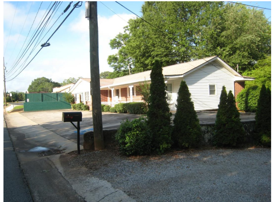
View of adjacent neighbor to the south at 14 Farmer Street
