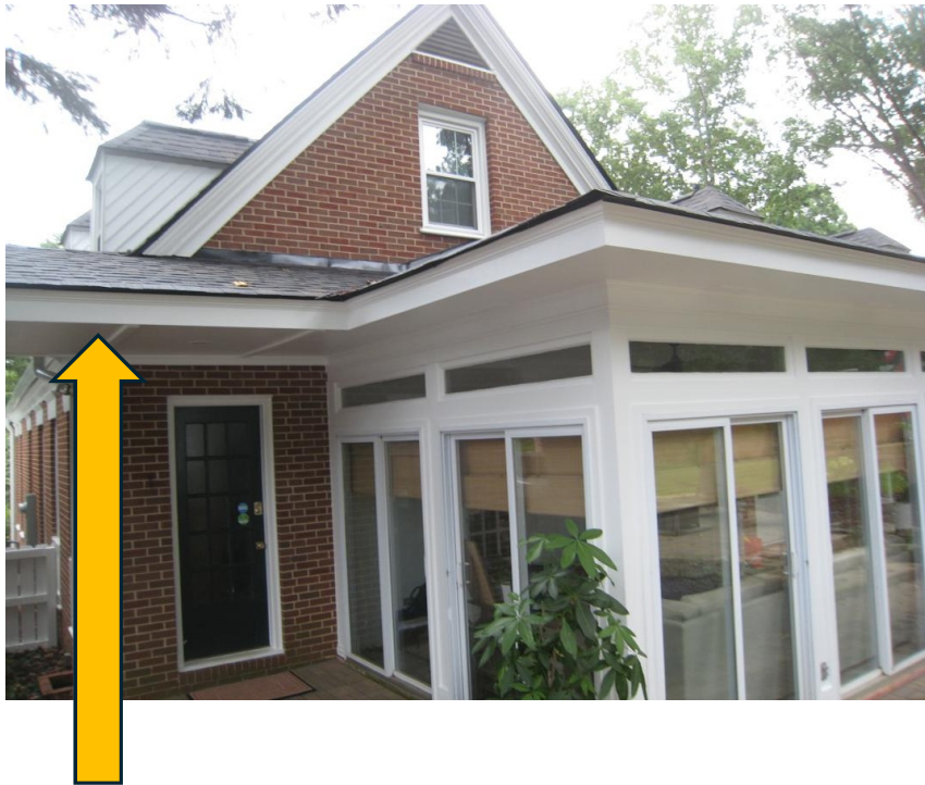
View of breezeway (shown with arrow) at its connection point with the house
