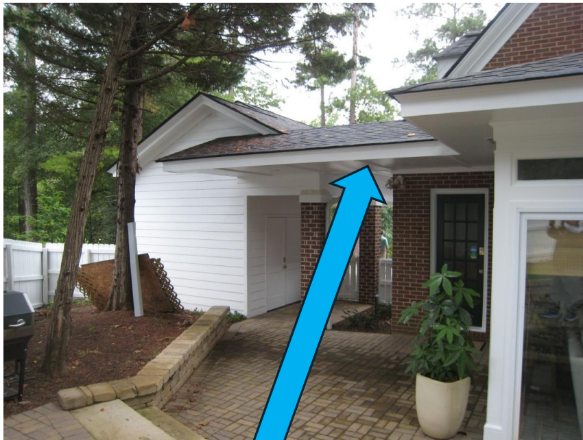
View of breezeway (shown with arrow) connecting house to the right and accessory building to the left
