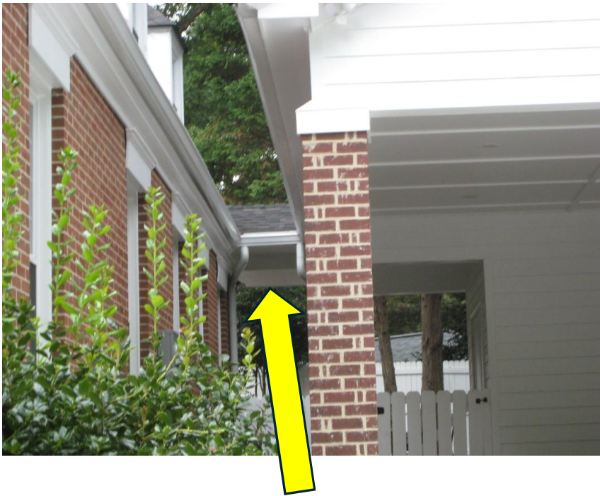
View of breezeway area (shown with arrow) as seen from the front carport area
