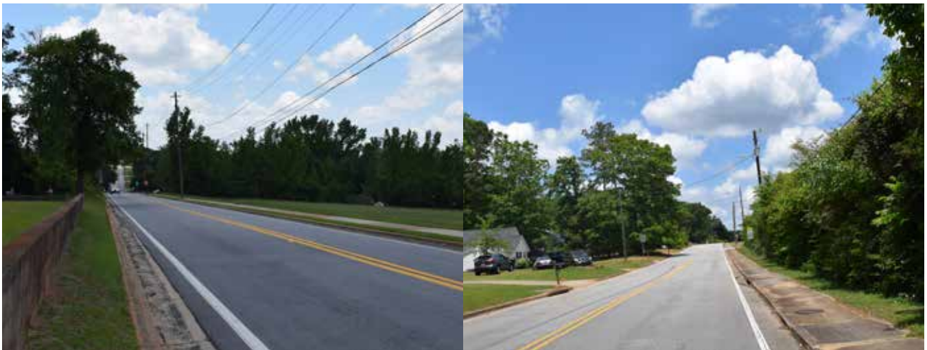
View to south of proposed mid-block crossing location on Boone Drive.
