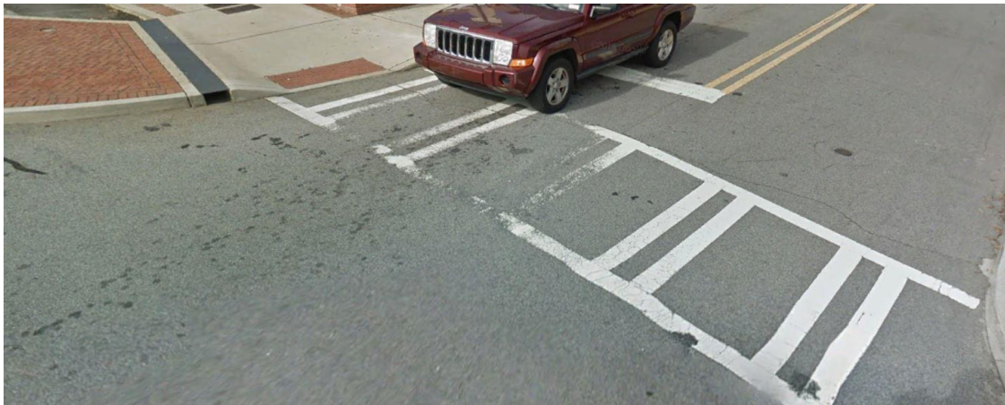
Picture #4 from Google Earth shows just how far back the stop bar is. I measured almost 30 feet from the stop bar to the travel lane edge.
