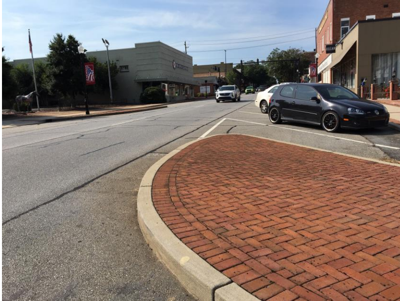
Picture #3 was taken near the end of the ped island where a vehicle's "nose" would be close to the inside travel lane. Notice that while sight distance is still somewhat hindered, it is better.
