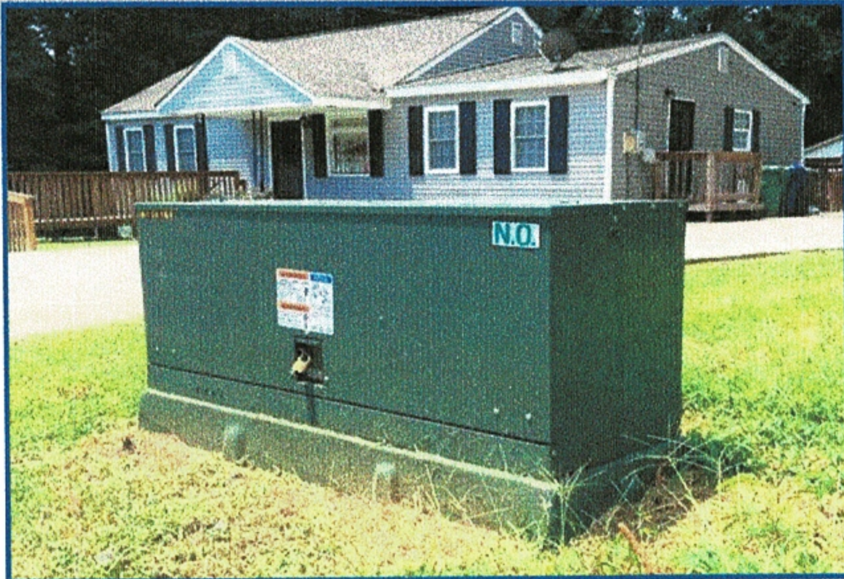
Three Phase Terminating Cabinet .85
