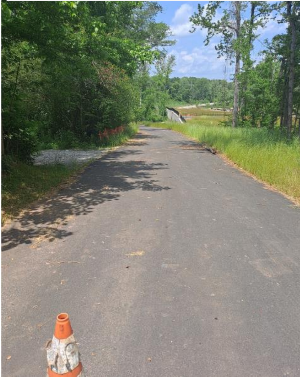
View of Emergency Access Road from edge of existing Pope Street paved area
