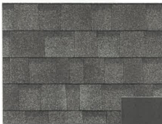
Architectural shingles & bronze gutters
