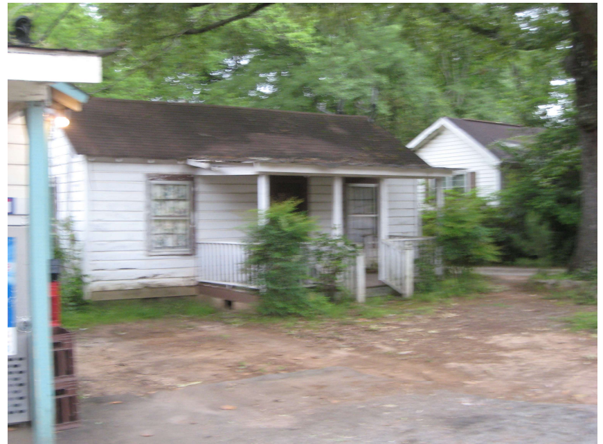
View of adjacent property at 68 Farmer Street
