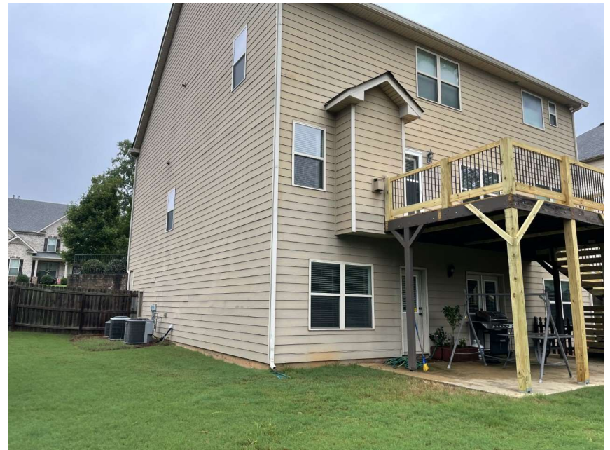
View of existing patio and side yard (looking towards Bryce Creek Drive)
