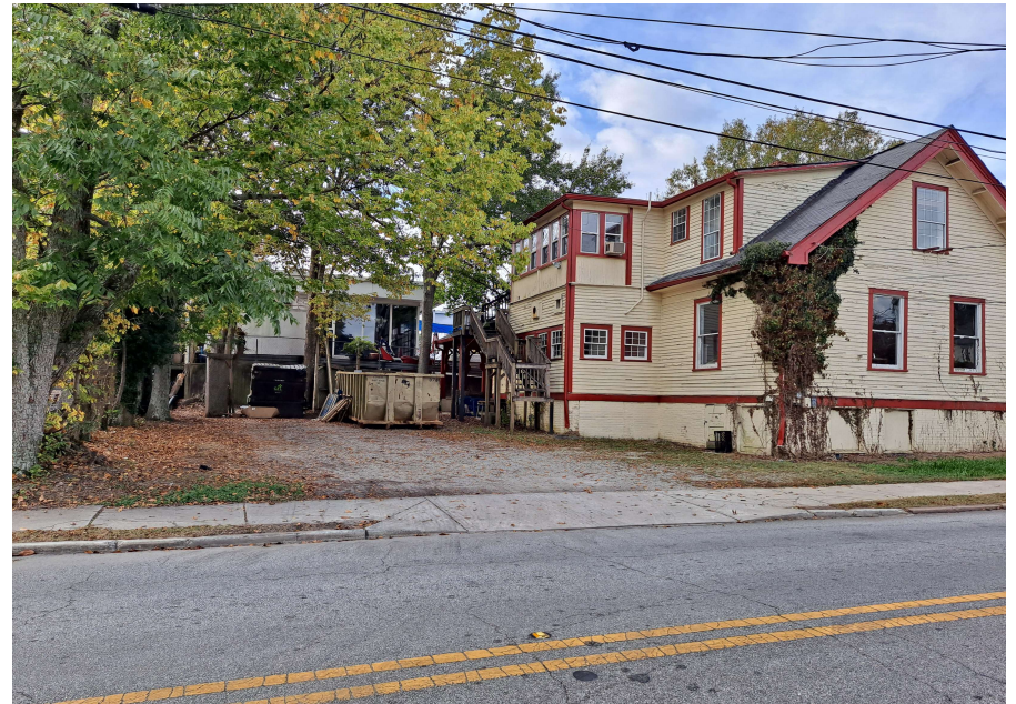
Picture of Subject Property Before Renovations from Wesley Street
