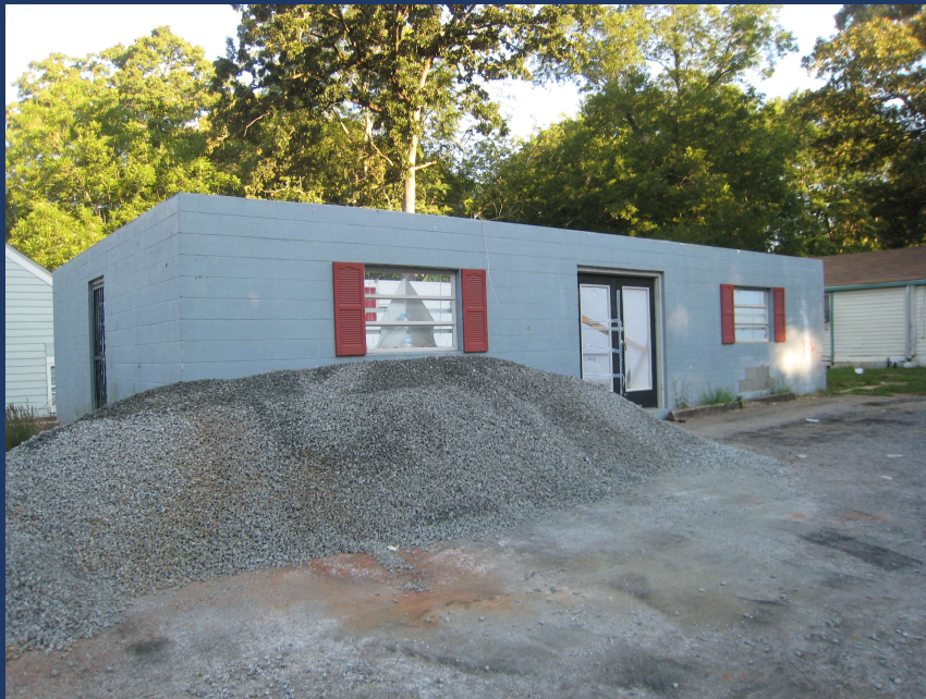
View of subject property from Farmer Street
