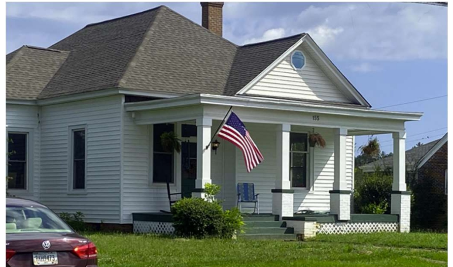
155 LaGrange Street (adjacent to subject property)
