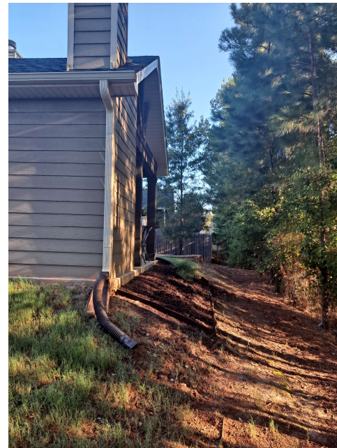
View of sloping area on the northern property line (adjacent to the proposed addition area)
