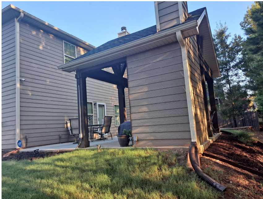
View of existing detached covered porch in rear yard
