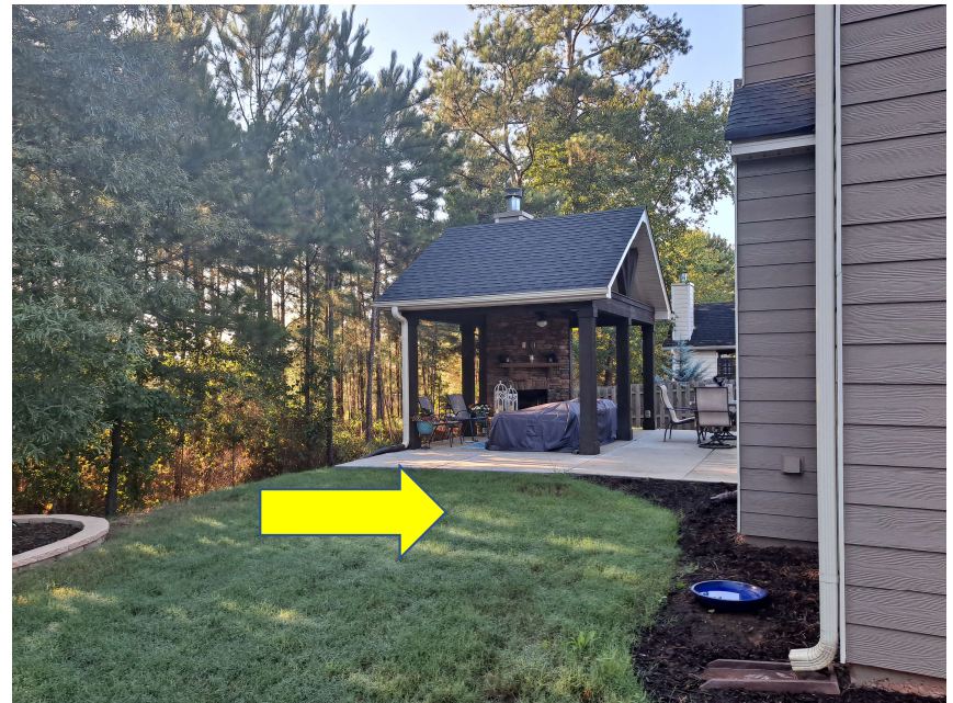
View of addition area in rear yard (actual addition area indicated by arrow)
