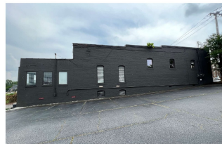
Existing Site Photos
