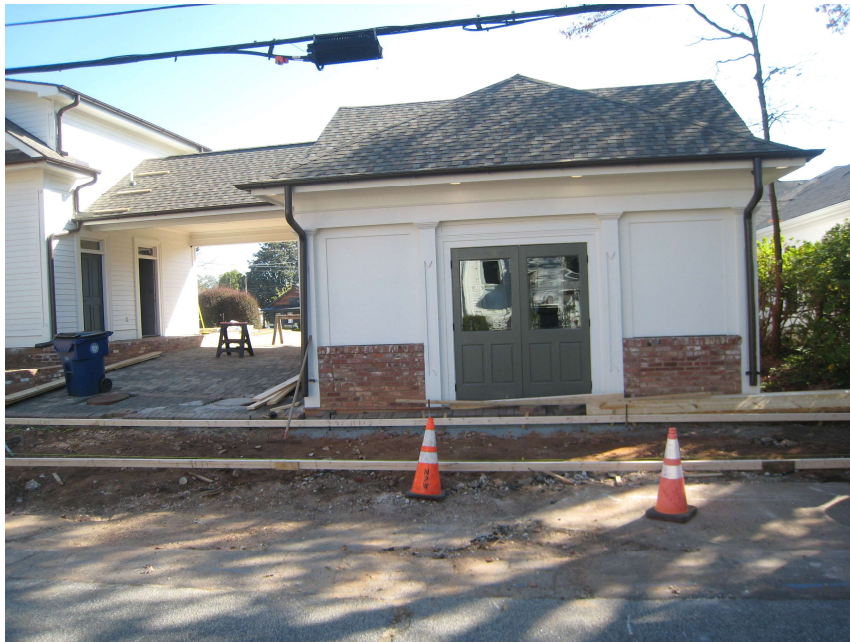
View of Front Elevation along Brown Street – Coffee Shop Building on right
