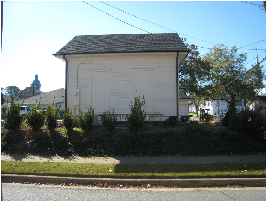
View of Left Elevation along Wesley Street
