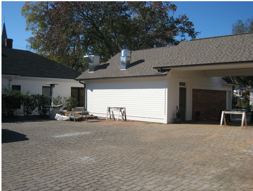
View of Rear Elevation (Coffee Shop Building)
