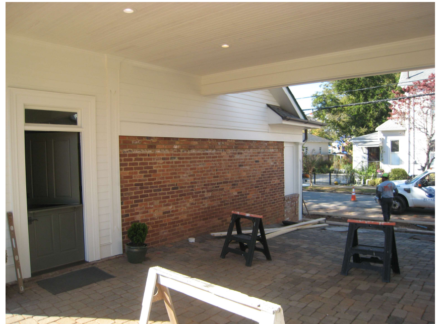
View of Interior Drive Area facing south towards Coffee Shop Building
