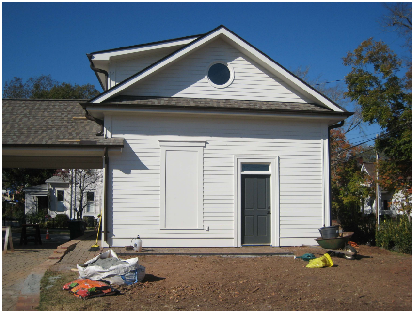
View of Rear Elevation (Storage/Toilet Building)
