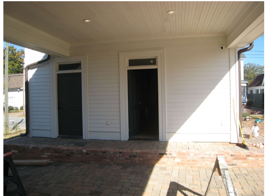
View of Interior Drive Area facing north towards Storage/Toilet Building
