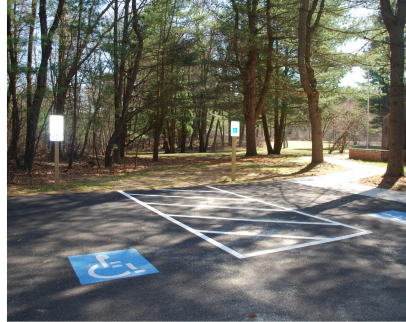
2,3,4: ASPHALT DRIVEWAY & ADA PARKING
