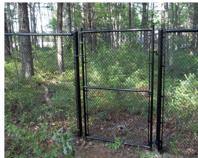
10,11: PERIMETER CHAIN LINK FENCE & GATE
