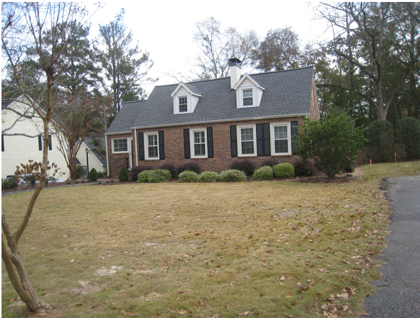
View of adjacent neighbor's front façade at 6 Parks Avenue
