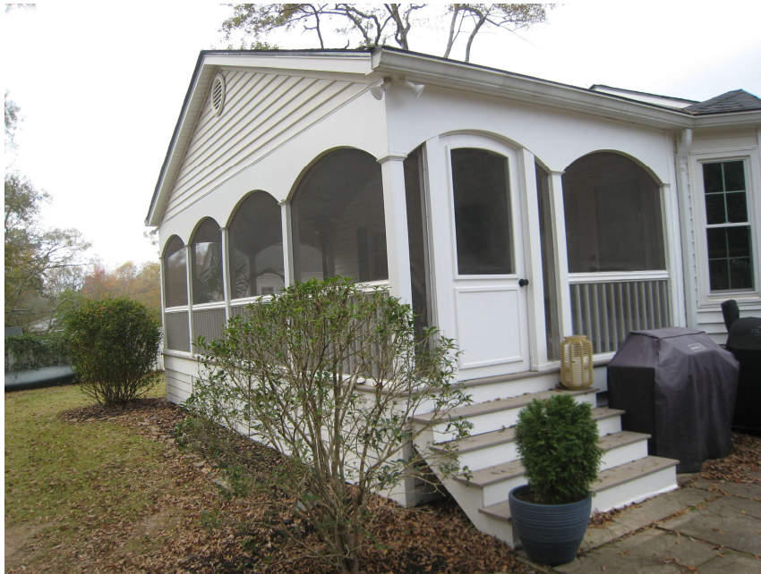
View of rear façade of subject property
