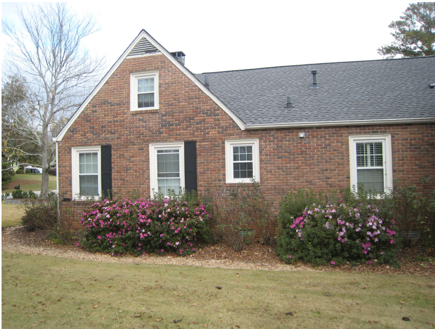
View of western side of neighbor's house at 6 Parks Avenue
