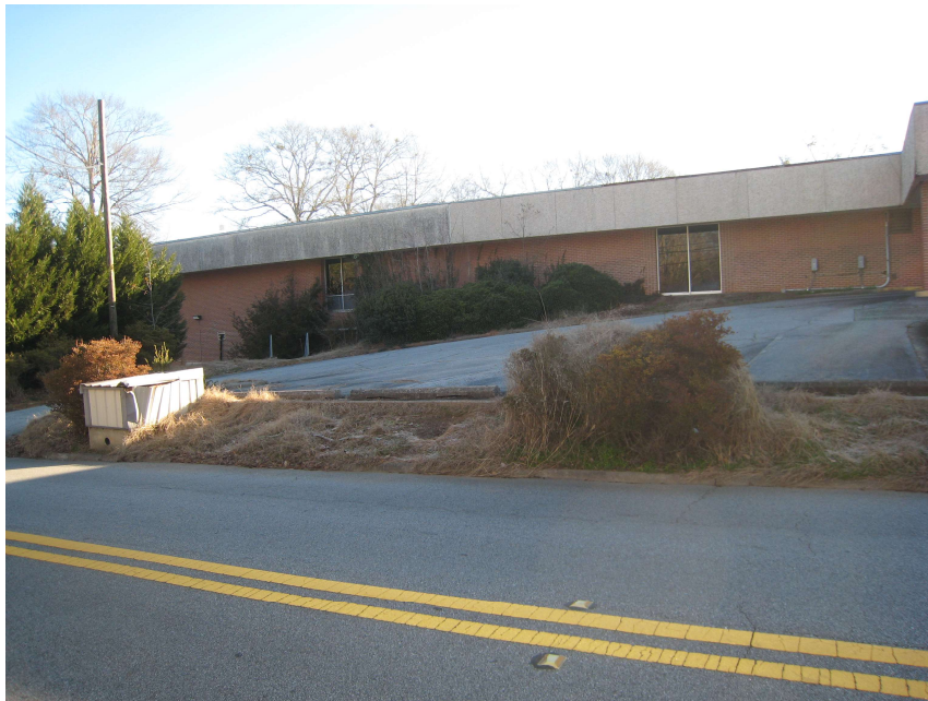
View of former Papp Clinic across Carmichael Street from subject property
