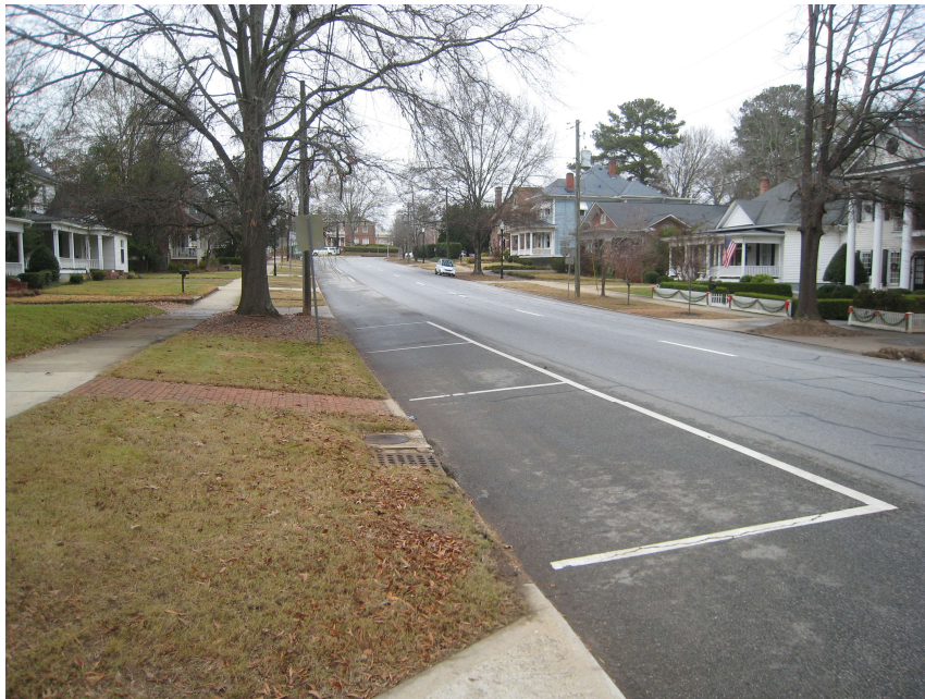
View to the north on Jackson Street
