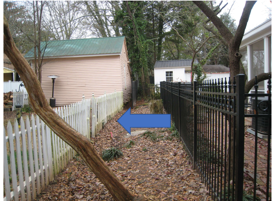
View of applicant's southern property line towards the rear of the subject property (blue arrow indicates existing water drainage area that flows to the front of subject property)
